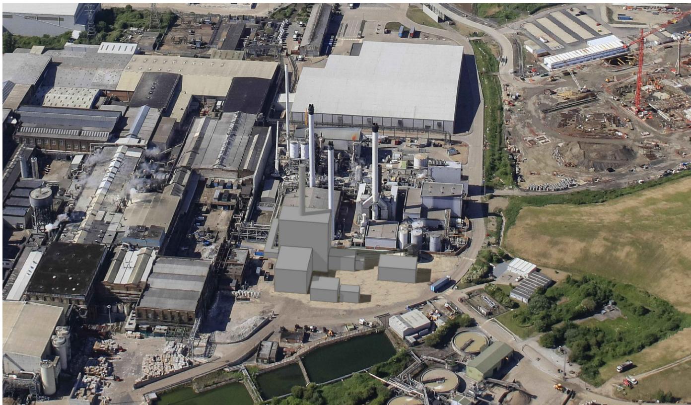
Figure 8: 3D visualisation of how it is intended K4 would look in the context of the existing Paper Mill site.
